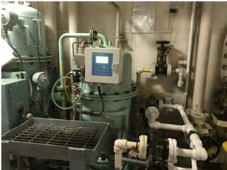
PHOTOGRAPH 38 Oily water separator - testing
